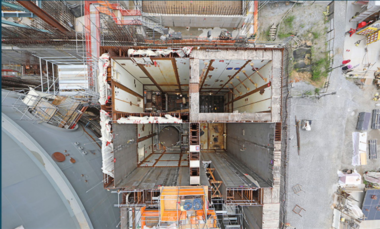
An aerial view of the Vogtle Unit 4 nuclear island looking inside the CA20 module.
