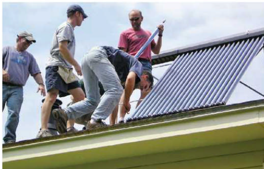
SOLAR SYSTEM: Members of a central New Hampshire initiative organize "energy raisers" that help neighbors install solar hot water systems.
